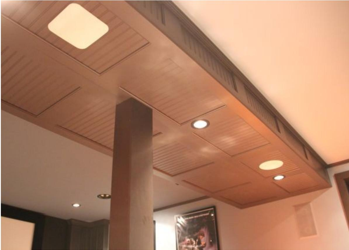
The rear height speakers integrated nicely with the soffit. Note the round and square grilles, both included with Noble Fidelity's L-65 mk II speaker.
